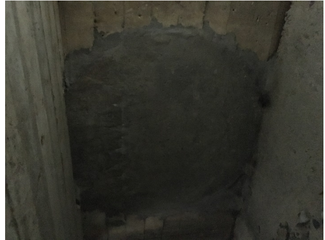
Figure 21: Concreted at 0.0m at MA70016043
